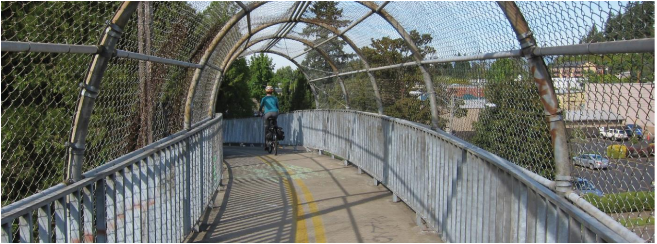
This overpass helps children cross a busy street at a midblock location.
